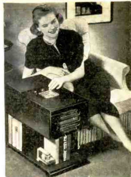
This very handy RCA "End Table" all-wave superhet has five tubes. Tuning range covers American "broadcast" stations, also the 49, 31, 25, 19 and 16 meter S-W bands, as well as Police and Amateur Calls.
